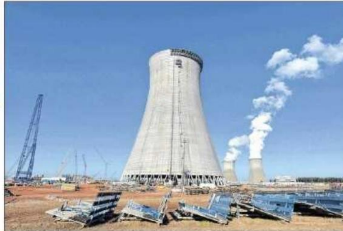
One of the two new cooling towers under construction at Plant Vogtle is shown in 2015 in the foreground of two existing towers. The construction of two new nuclear plants at Plant Vogtle has fallen years behind schedule. Georgia's Plant Vogtle is now the only nuclear plant under construction in the U.S. www.sandiegoblade.com
