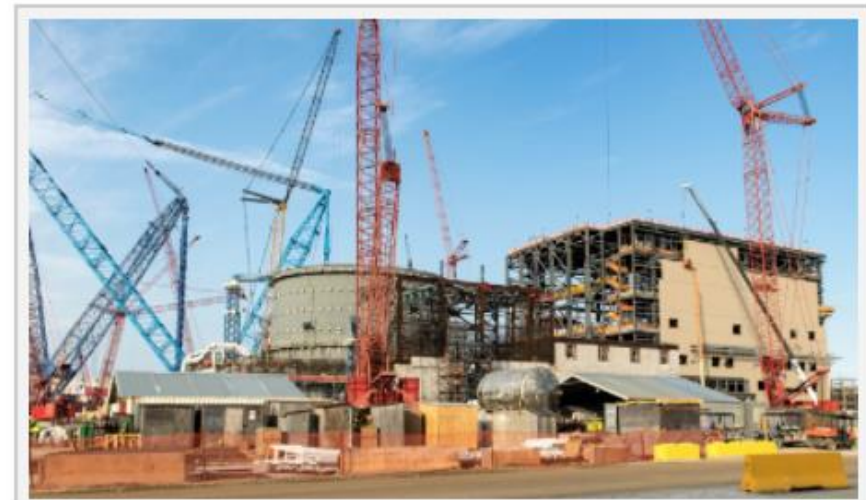
Photo of Vogtle Unit 3 in December 2017
