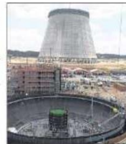
Expansion at Plant Vogtle will add enough new nuclear energy to power 500,000 homes. In this 2014 view, one of the two new cooling towers is seen in the background. MATT COOPER/MATT COOPER.COM
