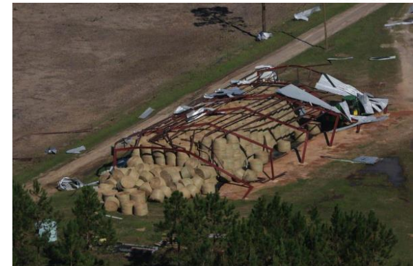
Farm damage from Hurricane Michael
