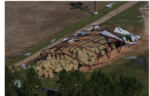
Farm damage from Hurricane Michael
