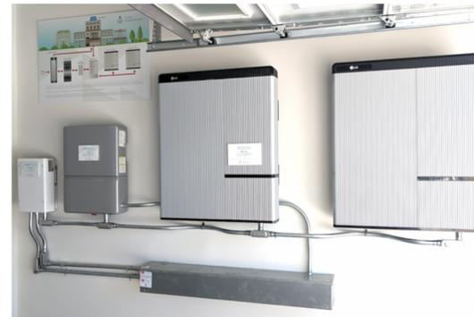
Garage with two 5 KW lithium-ion batteries, an EV charger, and a heat pump water heater
