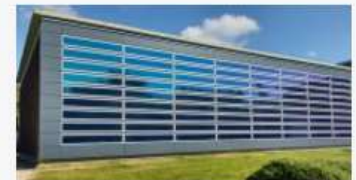
Solar active façade with HeliaFilm® at ENGIE labs
