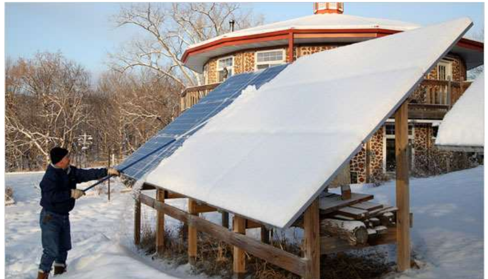
Solar Panels Covered in Snow
