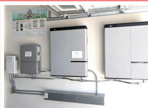
Garage with two 5 KW lithium-ion batteries, an EV charger, and a heat pump water heater
